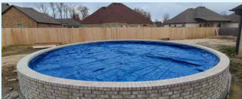
Stealth Cover Installed
